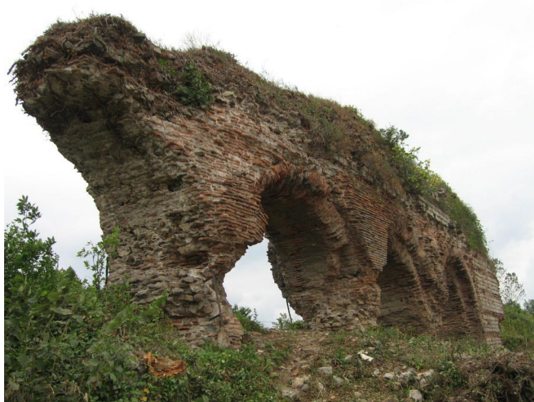
Figure 6-37: Remnant of Aqueduct Visible on the Surface to Ancient City of Teion 23
